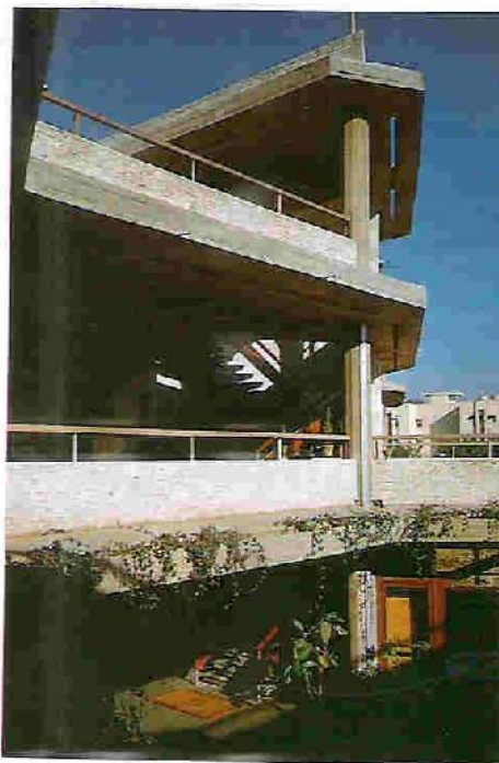
The staircase mummy and the water tank of the 7-8 o'clock block.
